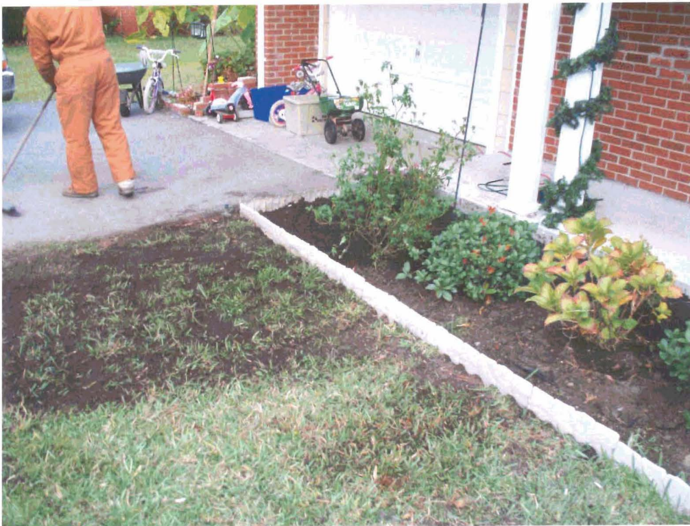
Picture 2: Location after removal of both tanks.
